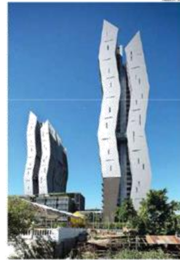
The 400-unit The Capers in Sentul East, was designed by RT+Q and instrumental in gentrifying the neighbourhood
